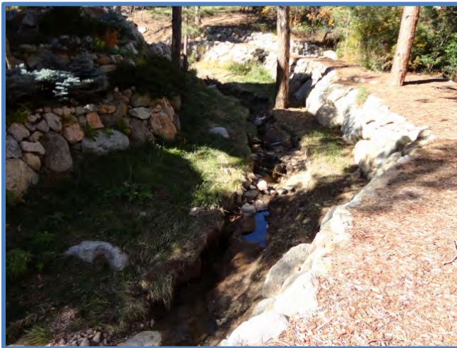
Photo 21D Northwest and 21E Southeast: Moderate erosion (3 – 4 feet deep) along section of drainageway upstream of CMP at Lot 3 [275 Stonebeck Lane]. Action: Repairs Recommended. Stabilize ground in drainageway between the boulder side walls.
