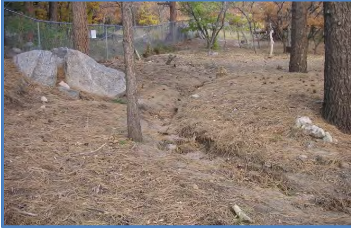
Photo 6B Northwest: The existing swale is too small to convey the flows from the upstream area. Action: Repairs Recommended. A swale and berm should be cut through backyard of Lot 10 to direct flows into the easement and towards the existing culvert at Paisley.
