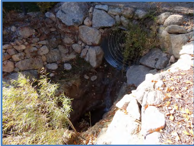
Photo 21C Northwest: Severe erosion at downstream end of private corrugated metal culvert in front of Lot 3 [275 Stonebeck Lane]. Action: Repairs Recommended. Stabilize ground at outlet of pipe.
