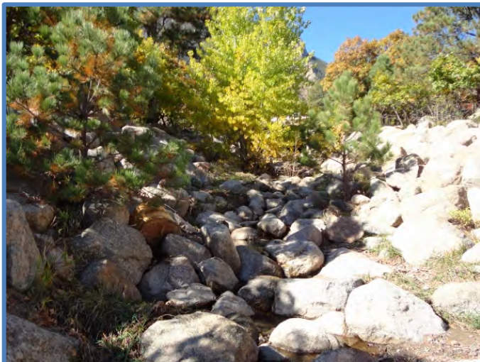
Photo 7A West: Small pine trees and a clump of aspens exist in the channel along the back of Lot 59 [5748 Adrienne Court]. Action: Monitor Condition. Monitor the trees and condition to avoid accumulation of debris along trees that would reduce the flow capacity of the drainageway.
