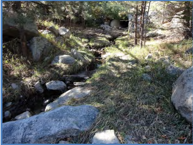
Photo 9A Southwest: Minor erosion in a few areas along Lot 19 [730 Paisley Drive]. Action: Good Condition. No action necessary.
