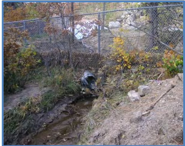
Photo 6C Southwest: A swale with sandbags and a culvert were installed upstream of the fence on the NORAD property. Action: Repairs Recommended. The swale downstream of the NORAD property should be protected from future erosion.
