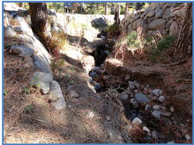
Photo 21D Northwest and 21E Southeast: Moderate erosion (3 – 4 feet deep) along section of drainageway upstream of CMP at Lot 3 [275 Stonebeck Lane]. Action: Repairs Recommended. Stabilize ground in drainageway between the boulder side walls.
