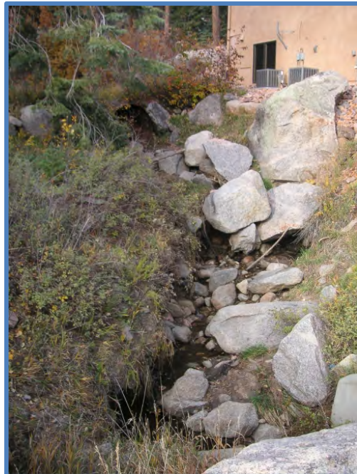
Photo 10A Southeast: Significant erosion downstream of the large boulders shown in the photo along the side slopes and bottom. Action: Repairs Recommended. Repairs to stabilize channel bottom and side slopes upstream of Paisley culvert.
